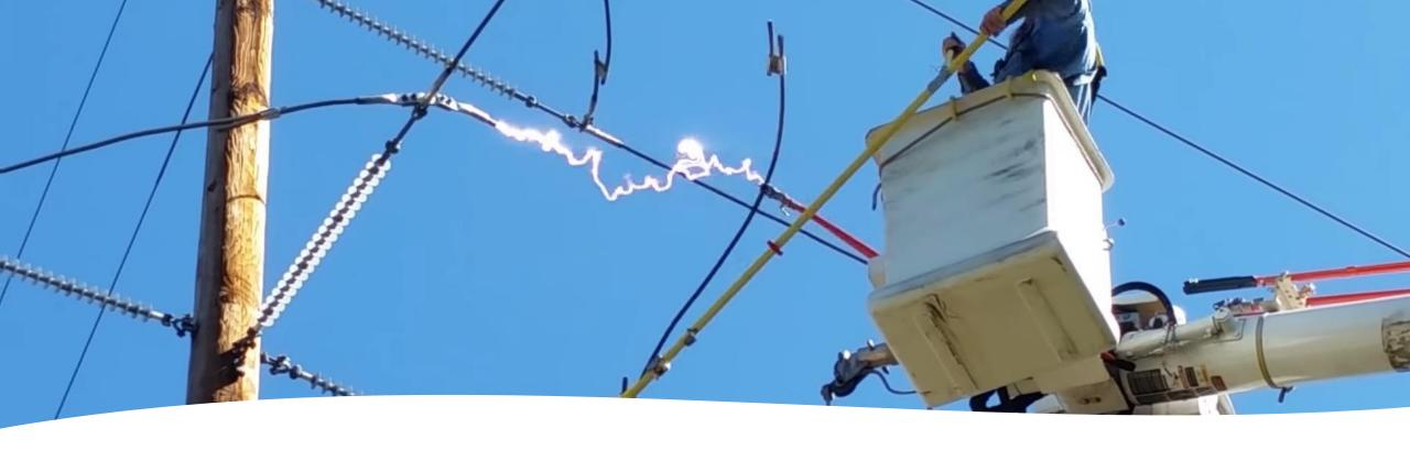
The GUS system works by reading the electric field which causes flashover. The system will alarm and then, if fitted with the optional interlock feature, issue a stop command at a preset "sensitivity", a multiple of the flashover distance.
